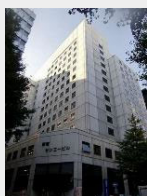
Shinjuku Sanei Building
